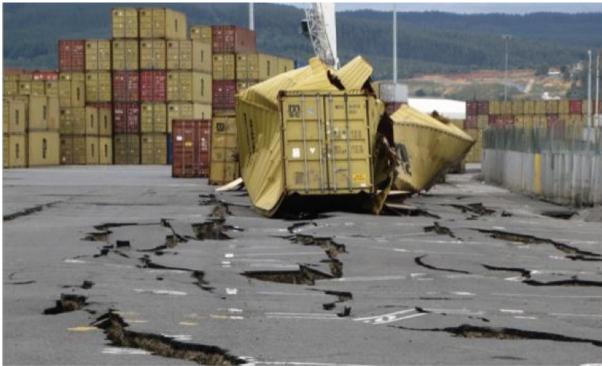
Damage to port due to liquefaction (photo: J. Bray)
