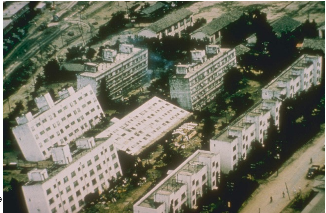
Damage to port due to liquefaction (photo: J. Bray)
