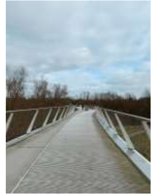
Living bridge on campus
