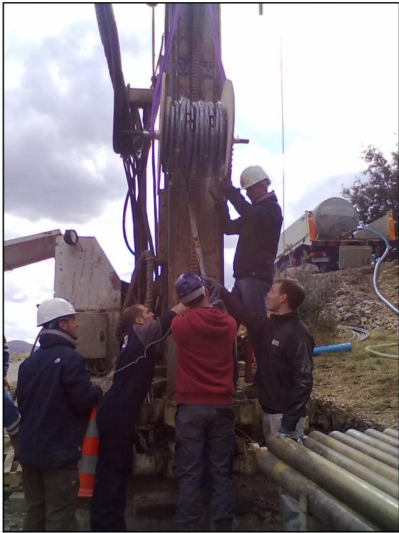
2 boreholes (60m, 1 cored)
